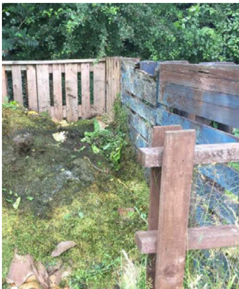
FODS Compost Area
